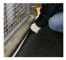
As soon as the primer coat has dried, the joint tape can be laid.
